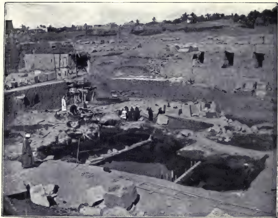
THE WORKS AT KARNAK IN JANUARY, 1906.
